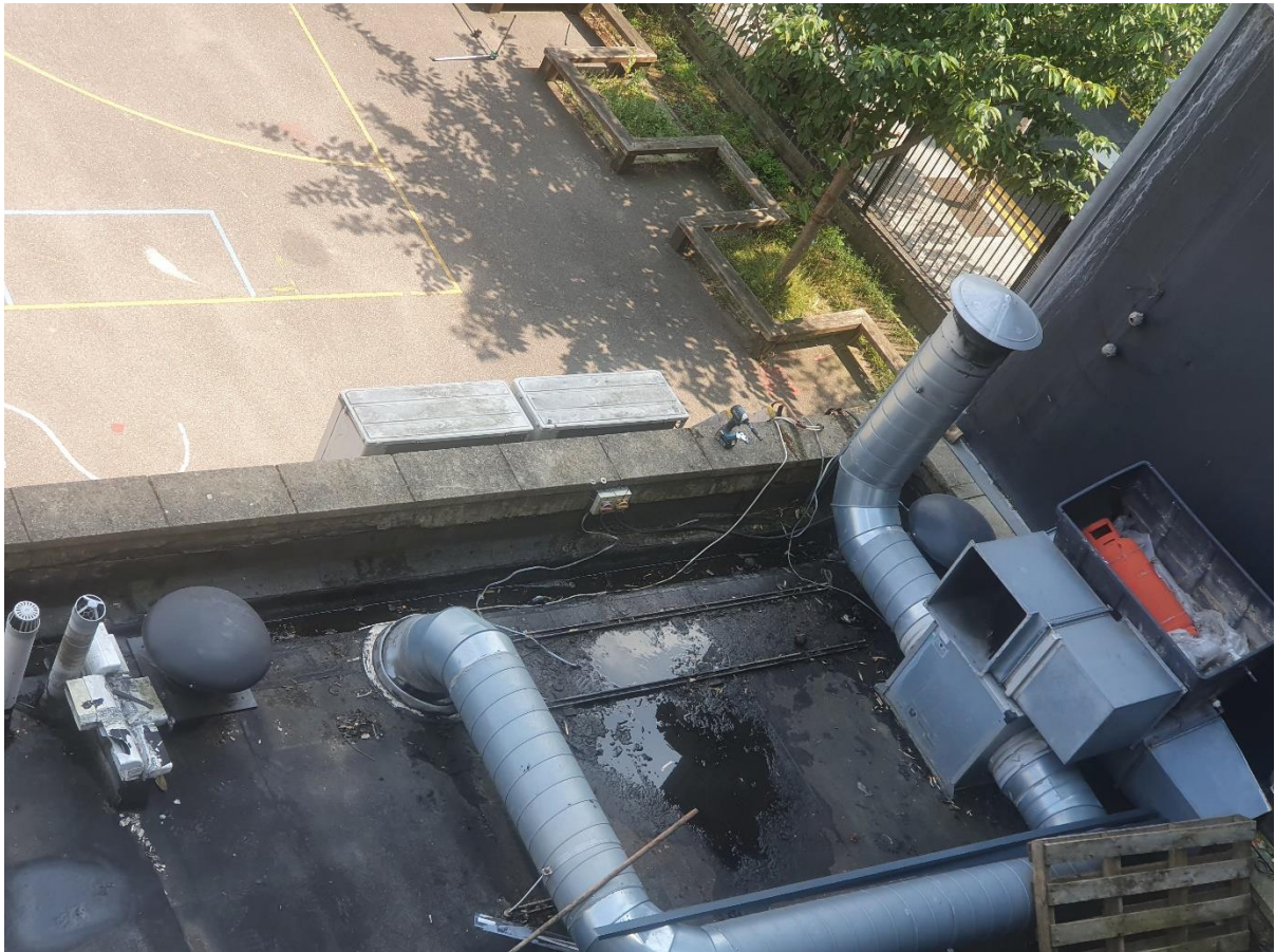
Figure 5 - Image showing new location of Simmons Bar's fans, to help with reduction of noise impacting residents.
