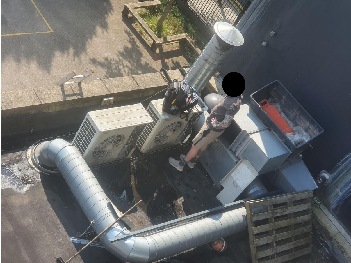
Figure 4 - Image showing initial location of Simmons Bar's fans, facing occupied flats.
