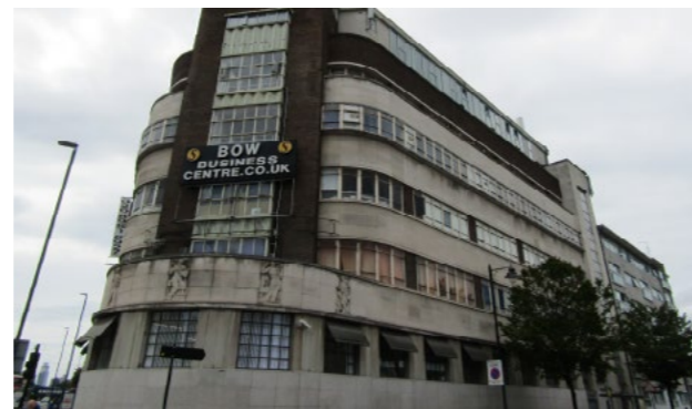
Fig. 15: Bow House Business Centre
