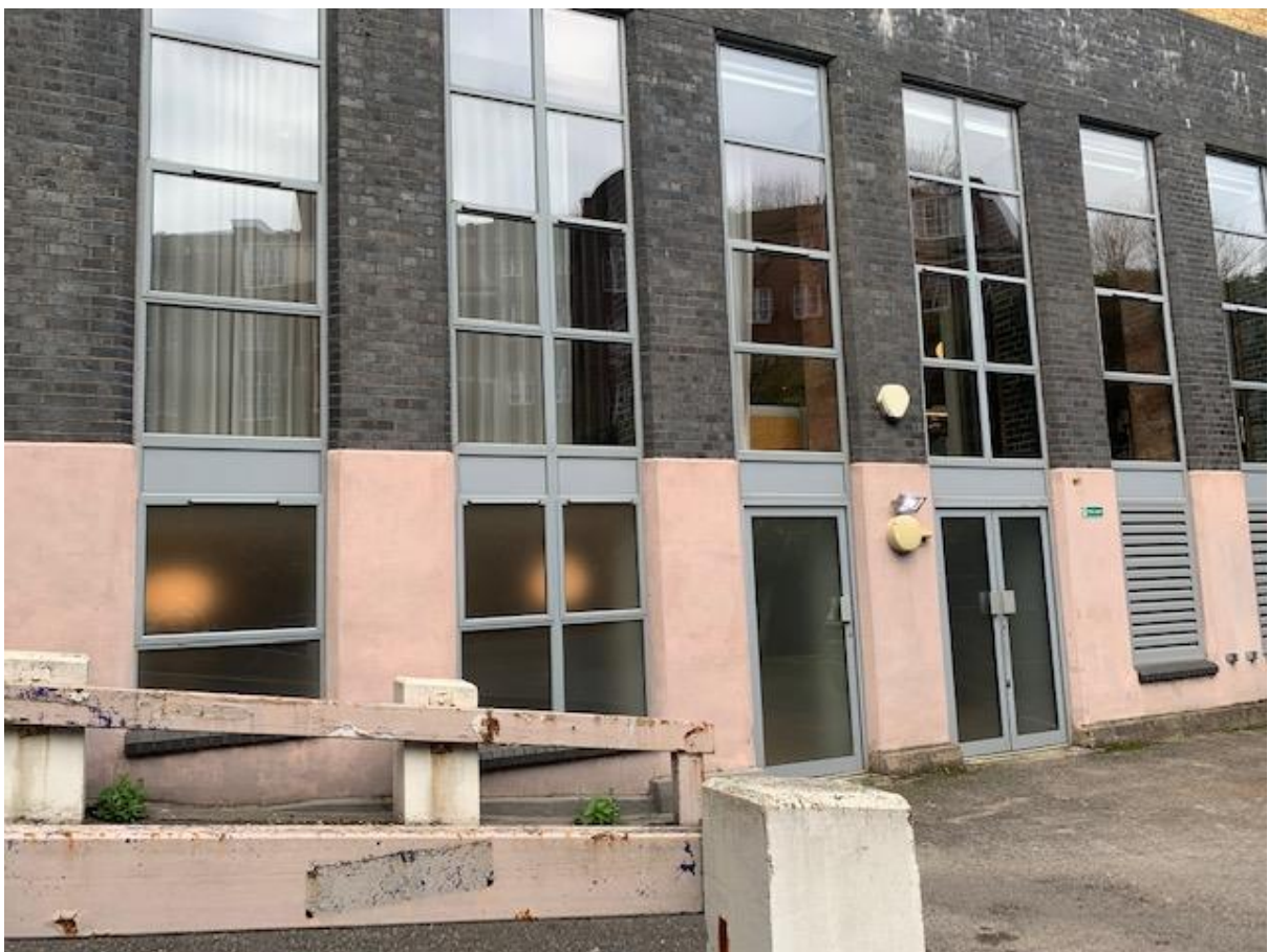
22 Calvert Avenue premises windows
