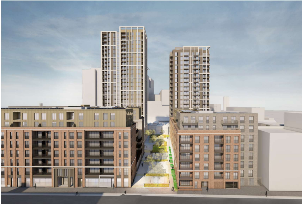
Figure 2: View of amended scheme from the east
