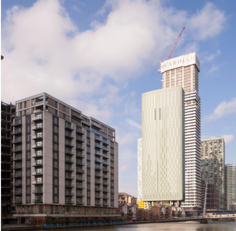
View looking west across South Dock
