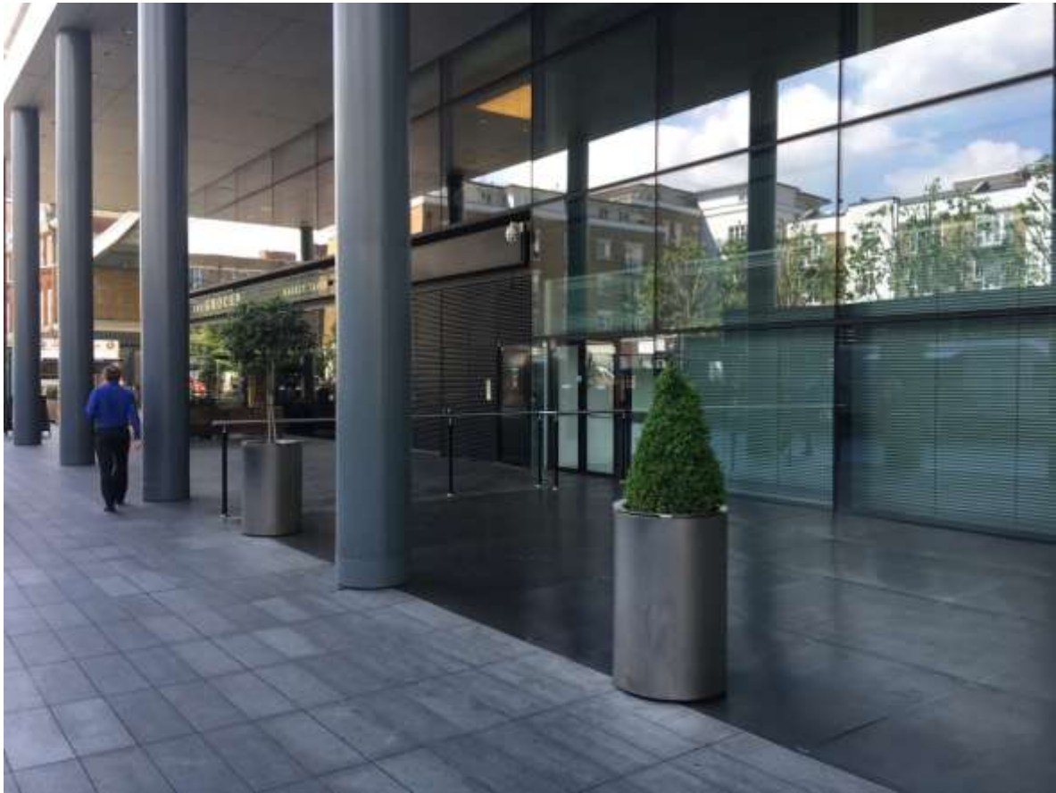
Image 4 – Lamb Street as existing (looking south-east)
