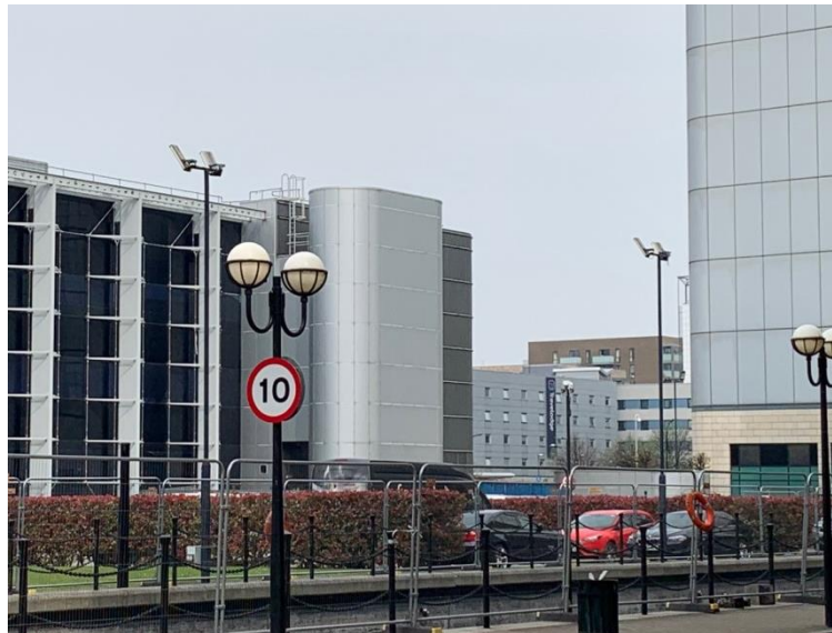
Figure 8: View of existing Travelodge hotel between East India Dock House (left) & Global Switch East (right)
