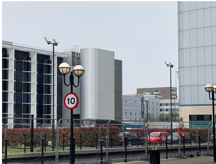
Figure 8: View of existing Travelodge hotel between East India Dock House (left) & Global Switch East (right)
