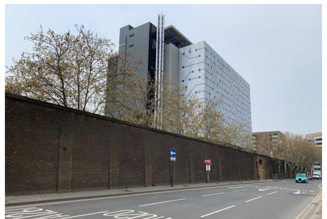
Figure 12: East India Dock Wall (TN2 data centre behind)
