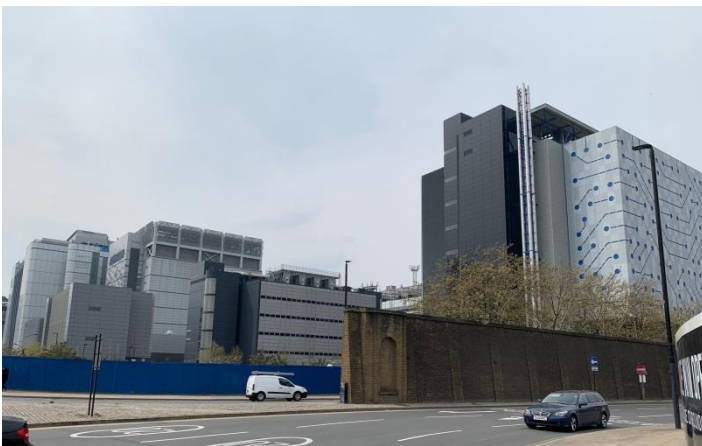
Figure 11: East India Dock Wall from Leamouth Road roundabout approach
