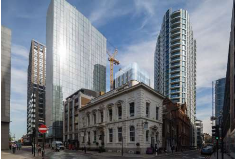
Figure 6: Photograph of existing site from corner of Alie Street and Leman Street with CGI image showing top of scheme (to left of crane) set above Grade II Dispensary. Built out serviced apartment hotel (1 Buckle Street) to left of crane in image an Altitude (to right).
