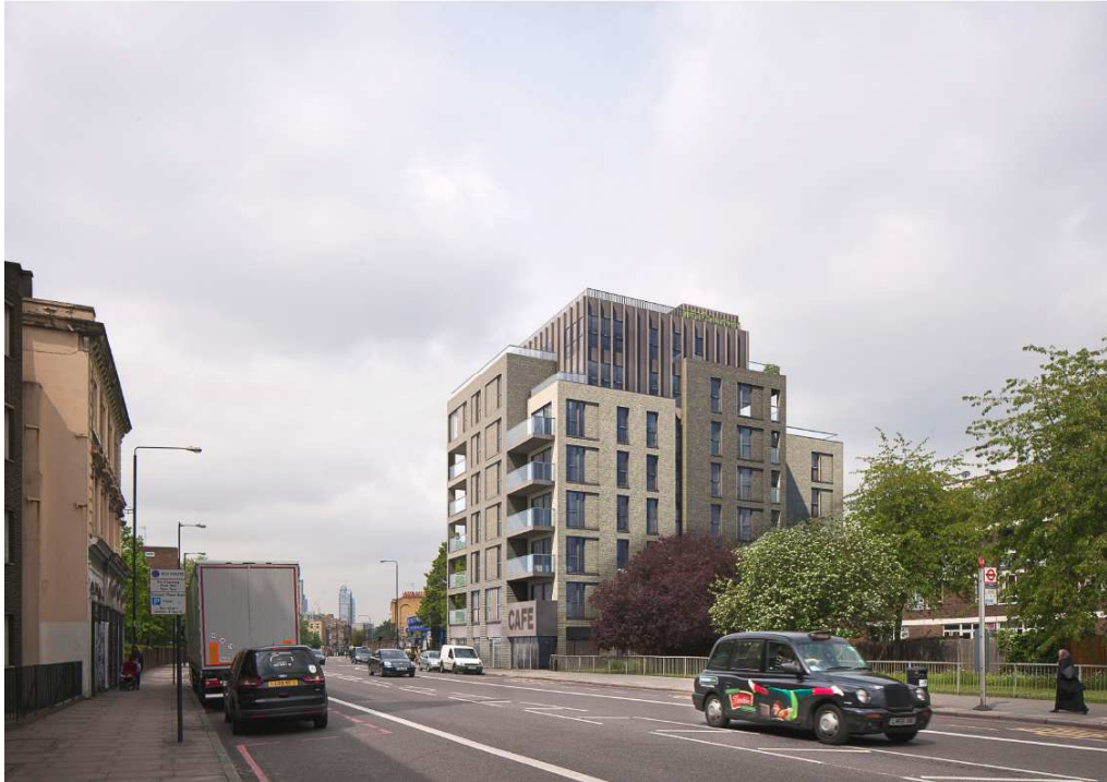
Figure 1 - View of the building looking west along Commercial Road
