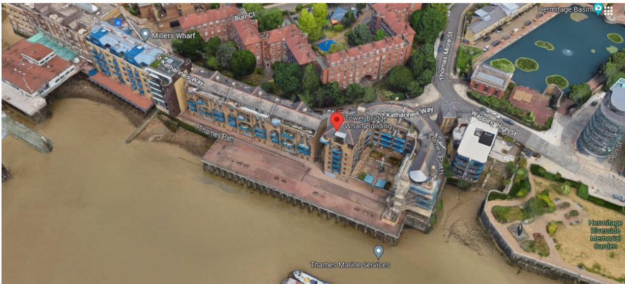
Figure 1: Aerial view of application site
