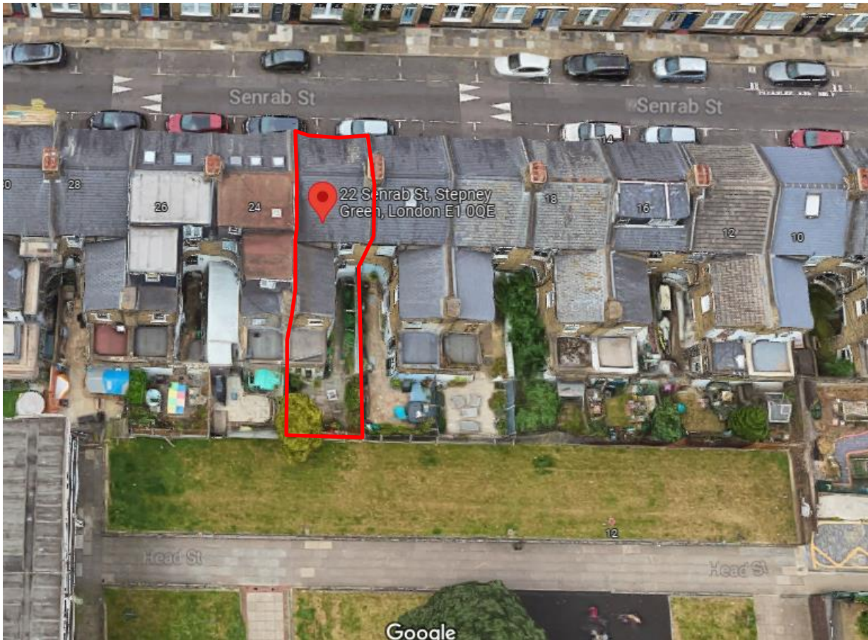
Figure 1: Aerial view of the site from the east
