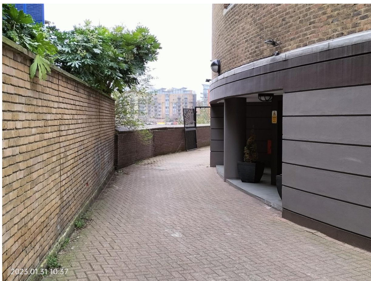
Figure 5: Eastern access gate to Thames Path
