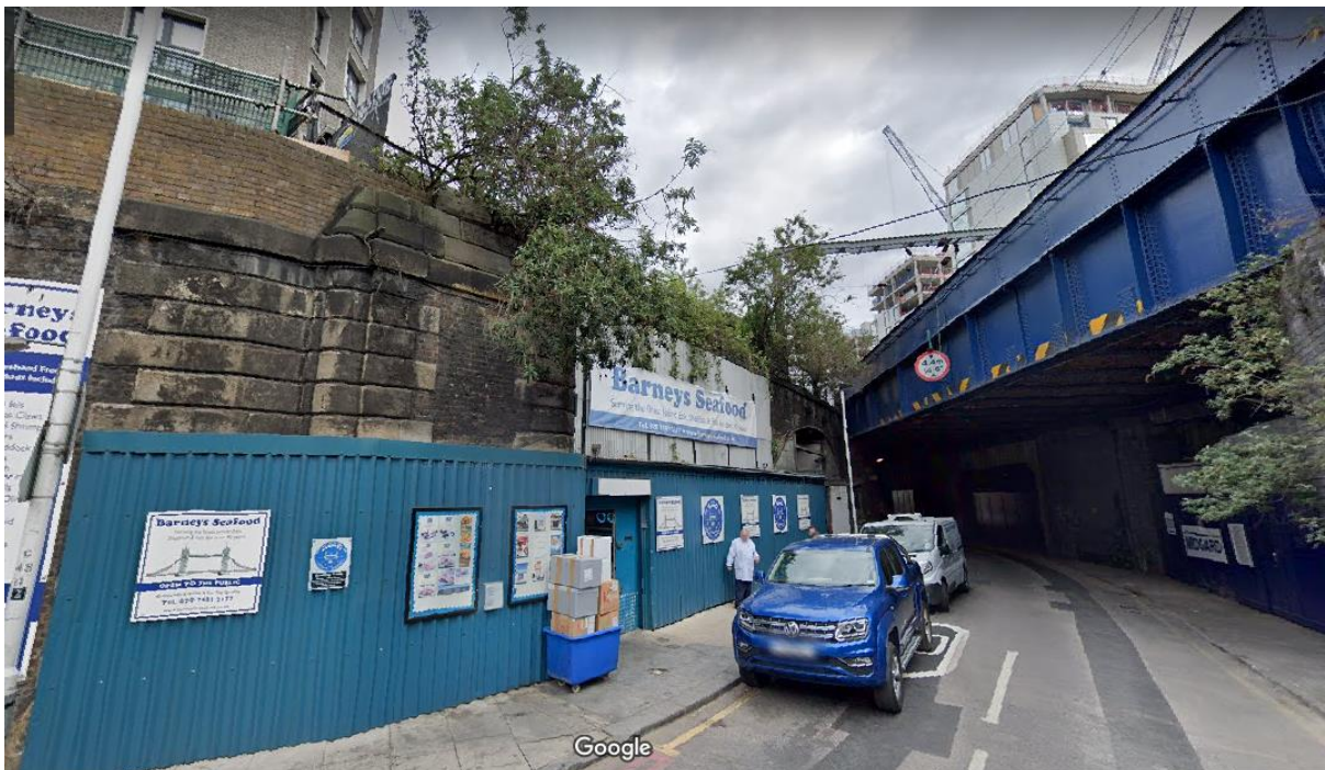
Figure B: View of the existing railway siding archways fronting Chamber Street
