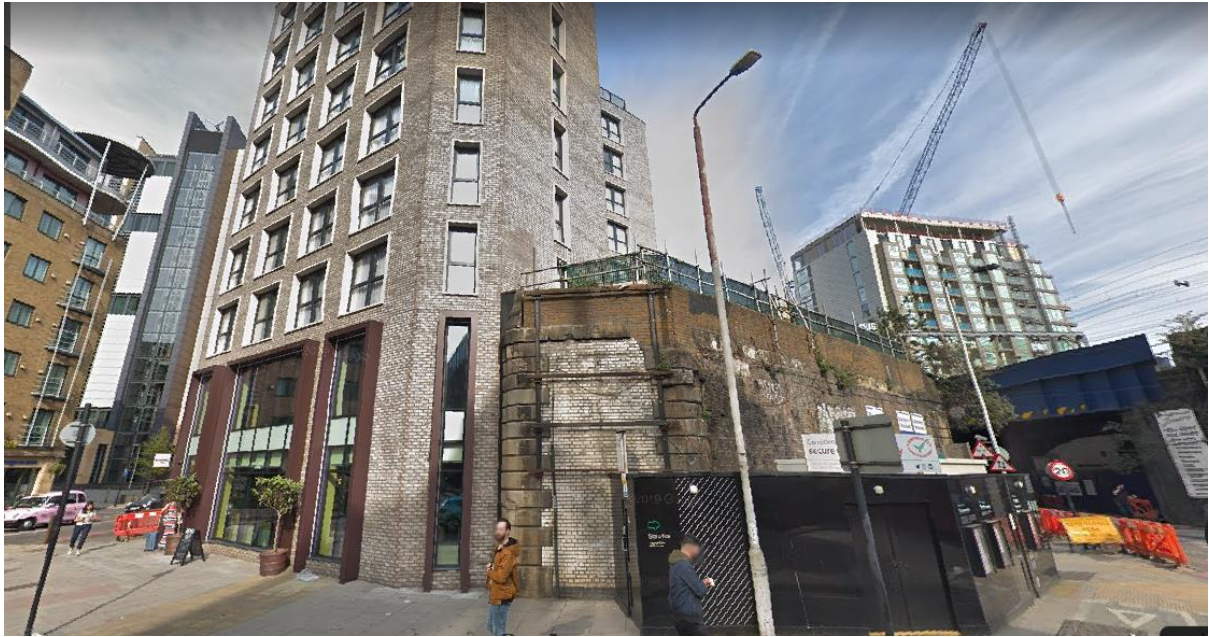
Figure C: View of the existing railway siding (right) and 99 Mansell Street and 31-33 Prescott Street development (left)
