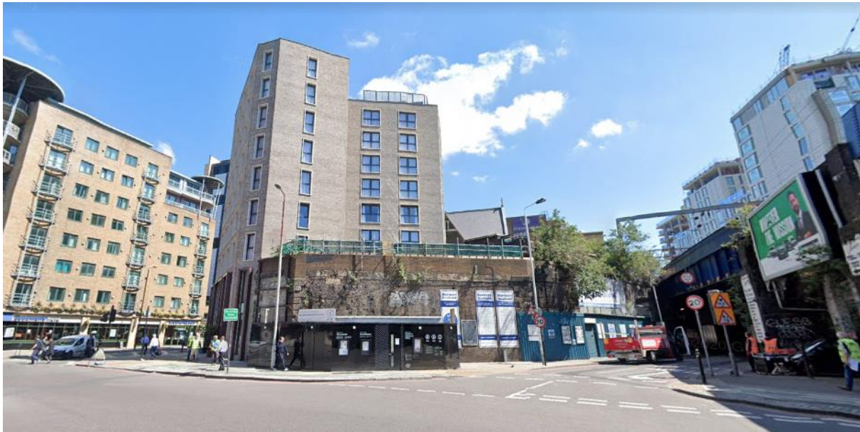
Figure A: View of the existing railway siding. The 99 Mansell Street and 31-33 Prescott Street development, and the rear section of the Roman Catholic Church of the English Martyrs roofline, can be seen to the rear of the railway siding.
