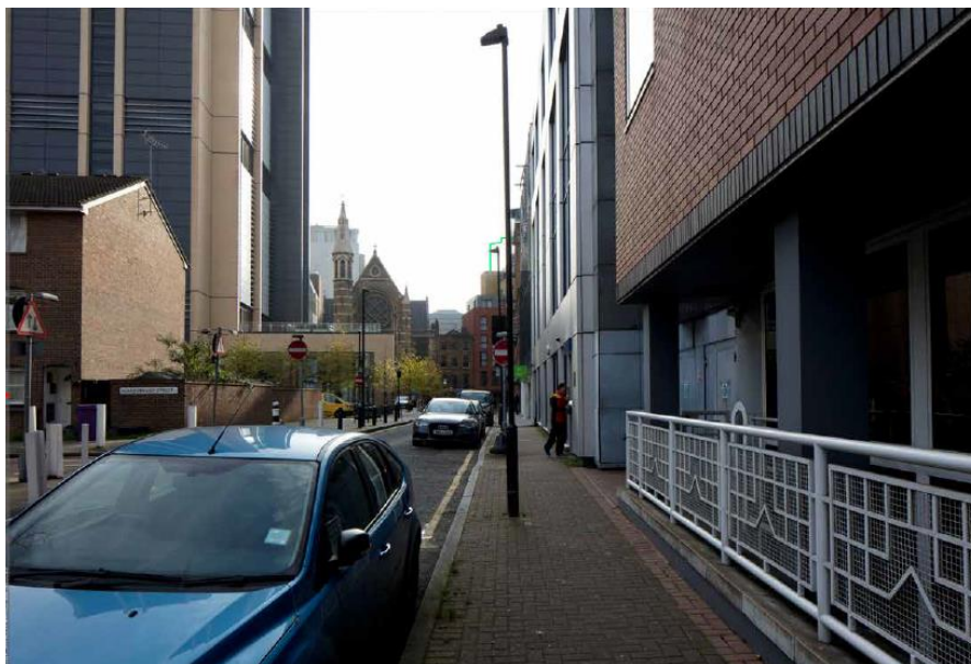
Figure 13: Verified View 4 – Proposed view south along West Tenter Street (west pavement). Proposed development: Green wire line
