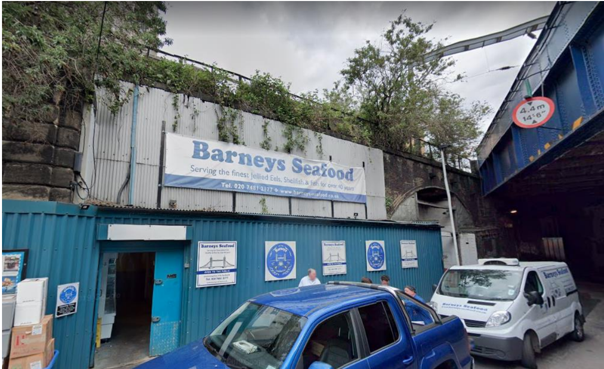
Figure 2: View of the existing railway siding archways fronting Chamber Street (left archway boarded up) and the previous site occupant, a seafood wholesaler
