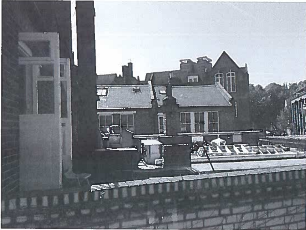
View from kitchen window to doorway of new dining room
