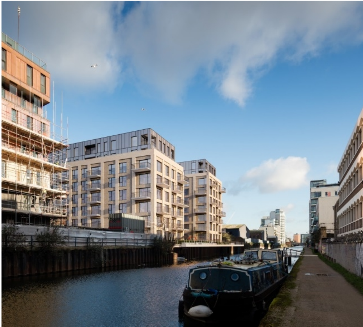
Figure 11 – Verified view from the canal towpath, looking north-east
